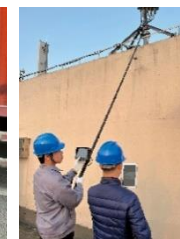
constructure inspection (WIFI real-time image transmission)
